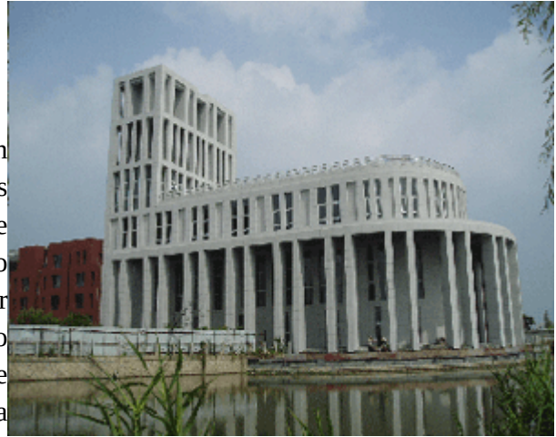
Fig. 9 : Anting Church (under construction).
