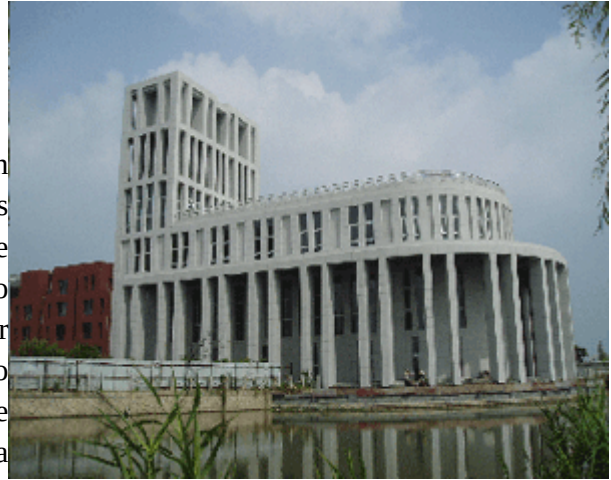
Fig. 9 : Anting Church (under construction).
